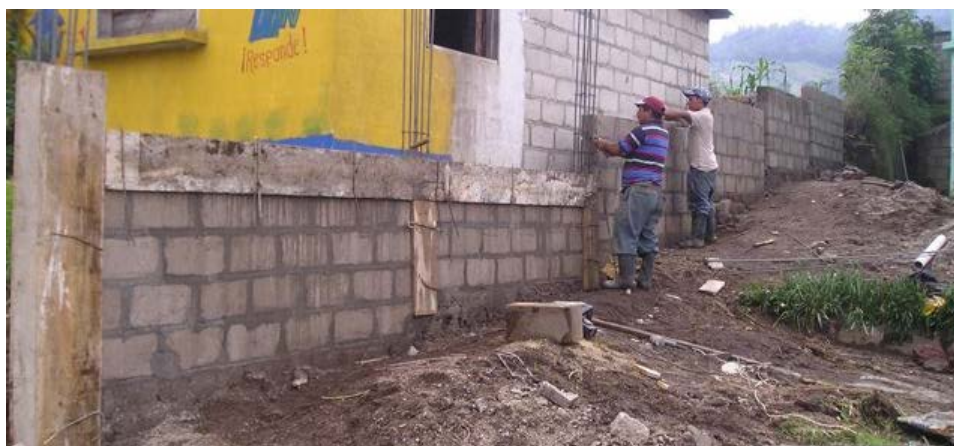
New retaining wall shown here under construction mid-June 2010.
